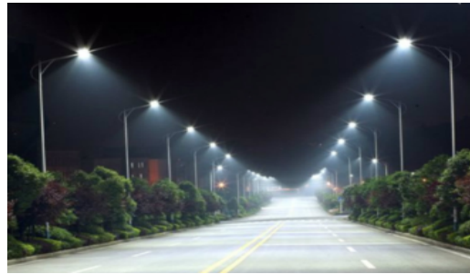
50,000 street lights and 6000 sign lights
